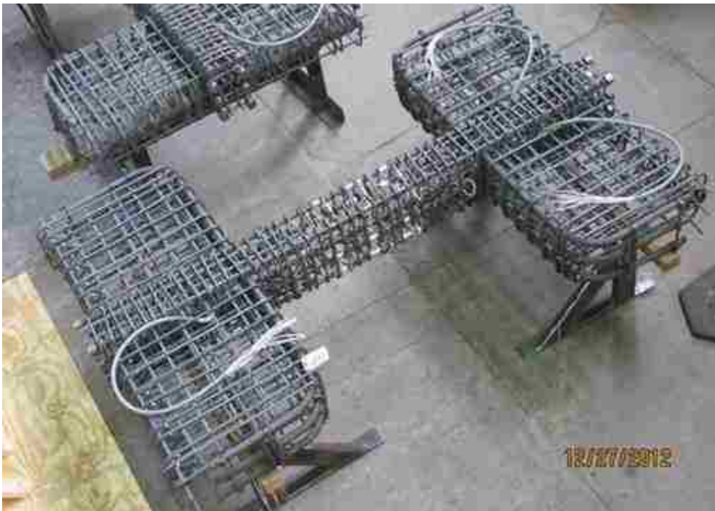
Figure 3-36: Reinforcement of TS02
