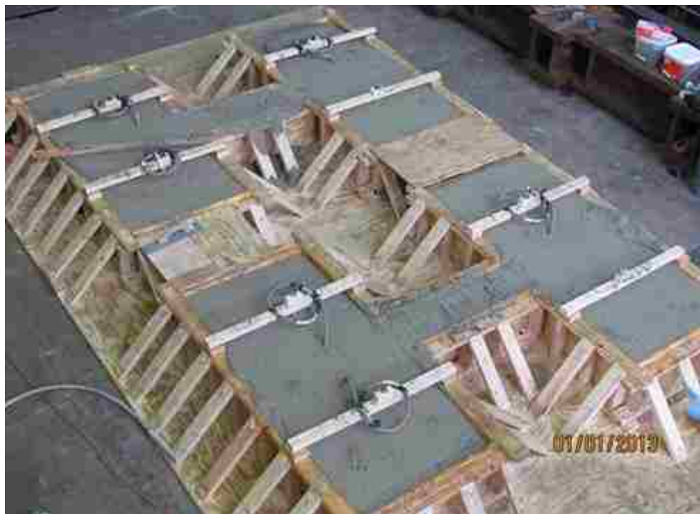
Figure 3-47: Concrete casting of test specimens
