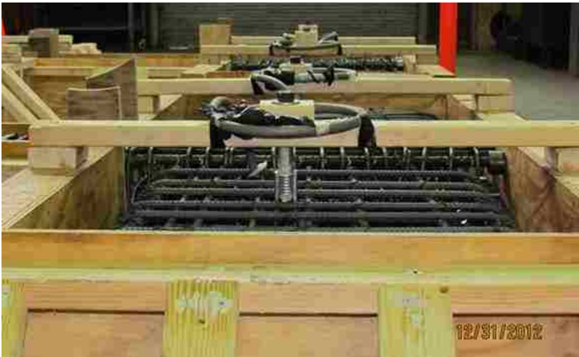
Figure 3-42: Lifting inserts installation
