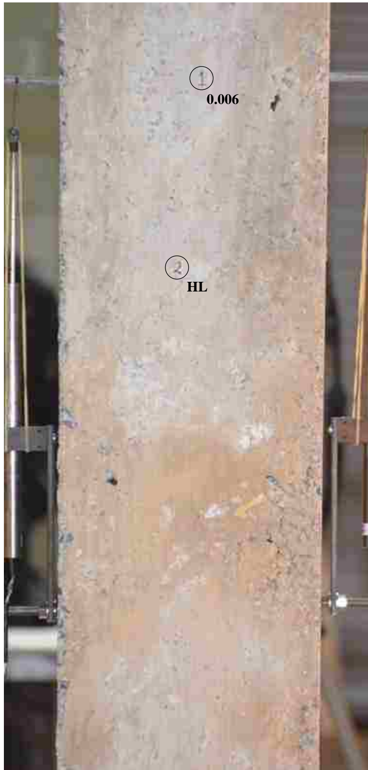
Figure 4-90: Cracks on west face of TS02 at Load Step 07
